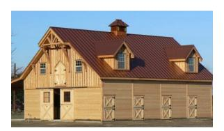
Each Loc-Rib™ panel snaps securely over the adjacent panel, eliminating the use of unsightly exposed fasteners. Loc-Rib™ panels are a snap to install and our design ensures that they stay locked without a need for "extras," such as seaming tools, washers or clips!
