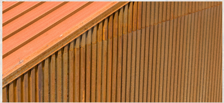
Redfox Commons, Portland, OR Featuring 16" MS200™ Roof Panels & Custom Contour Series™ Wall Panels
