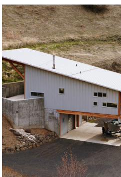
Rusteel Plus™ (A606) general appearance prior to being exposed to the weather
