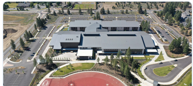
CALDERA HIGH SCHOOL • BEND, OR — standing-seam metal roof by Taylor Metal Products
